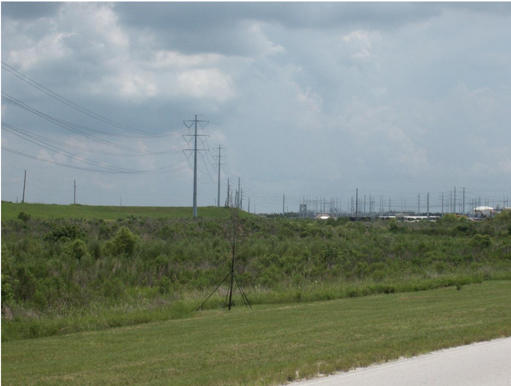
Utilities (8300) - Ground photo
