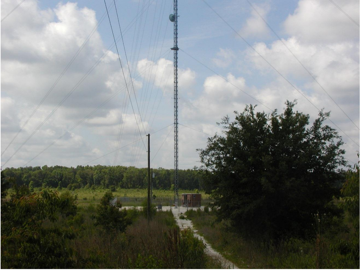
Communications (8200) - Ground photo
