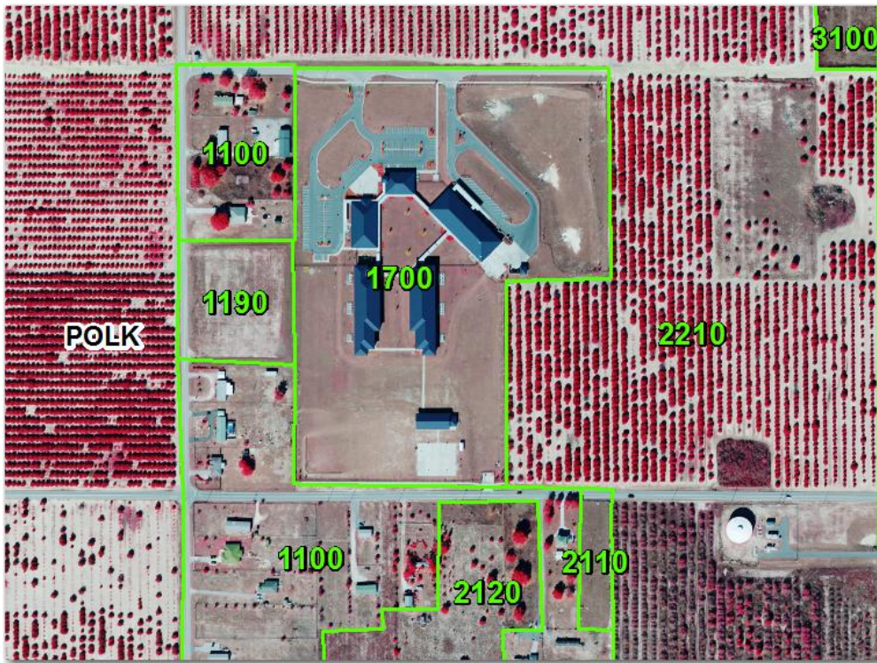
Low Density under Construction (1190) - Color Infrared aerial photograph
