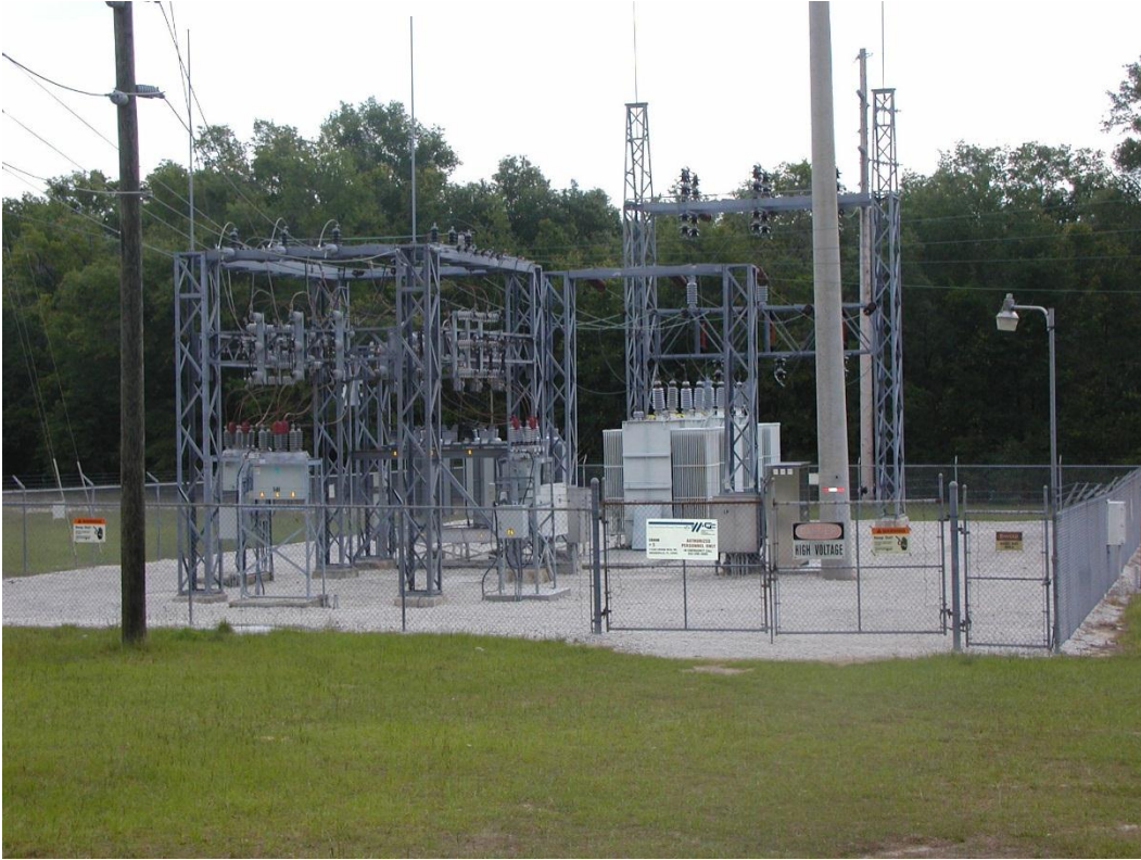
Utilities (8300) - Ground photo
