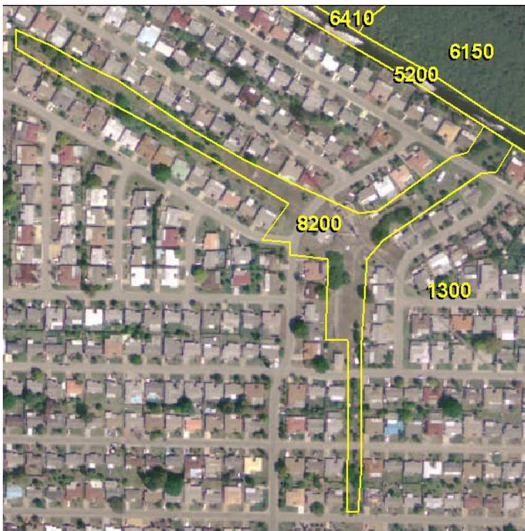
Communications (8200) - Natural color aerial photograph
