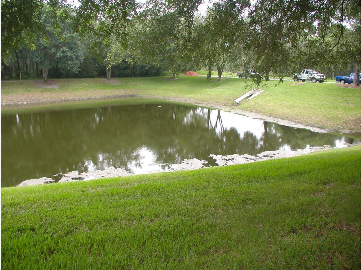
Water - Reservoirs (5300) - Ground photo
