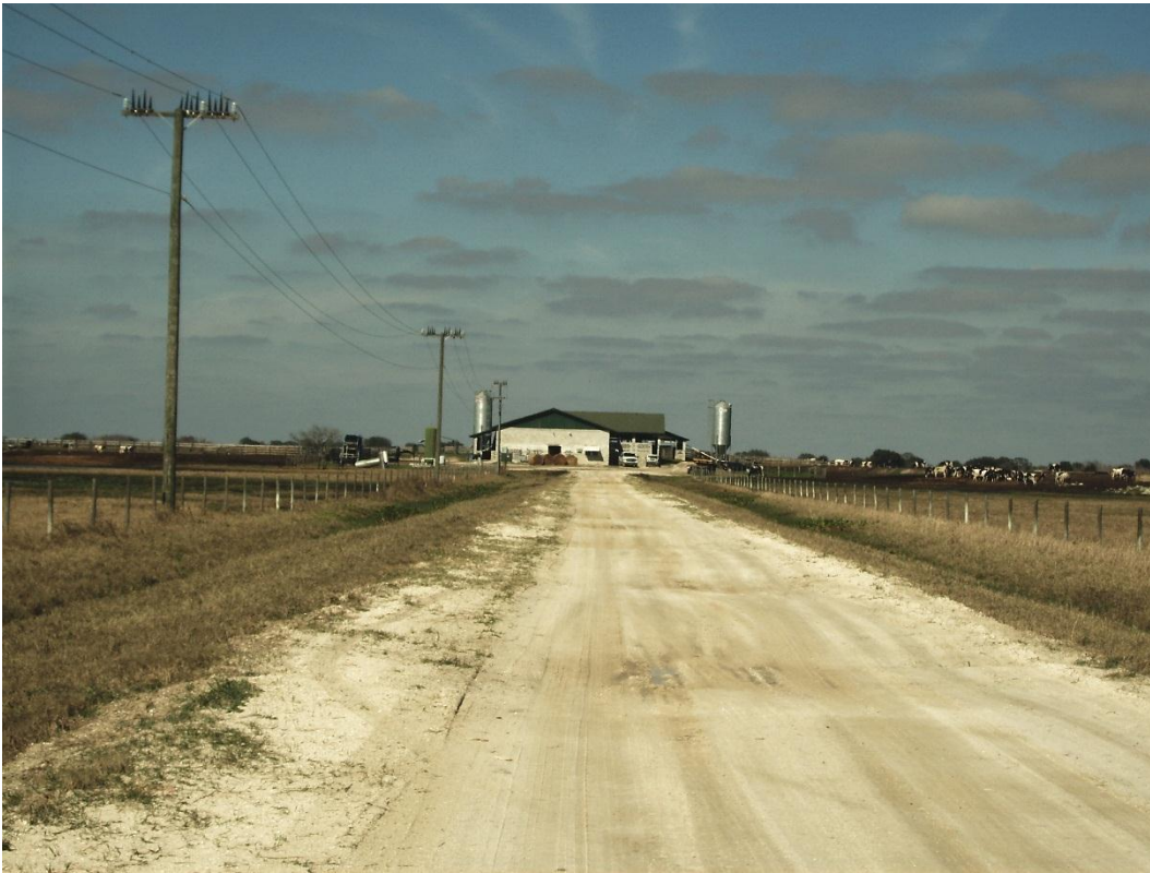
Feeding Operations (2300) - Ground photo
